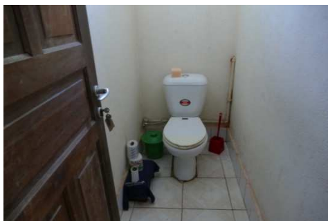
Figure 17 - Pose de WC
